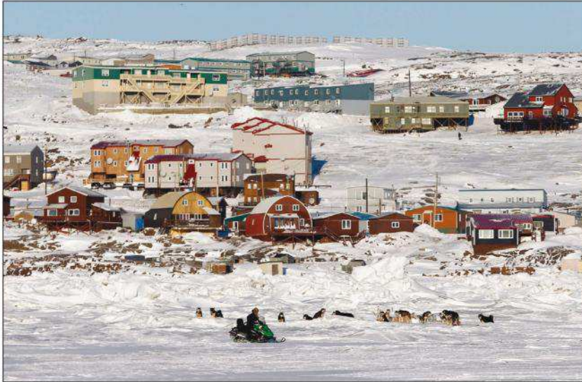
In Iqaluit, in the Canadian territory of Nunavut, homes are sinking into the warming earth.
